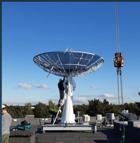
Parabolic dish Downlink (4,9-meters)
